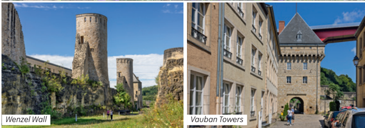
The Three Towers
